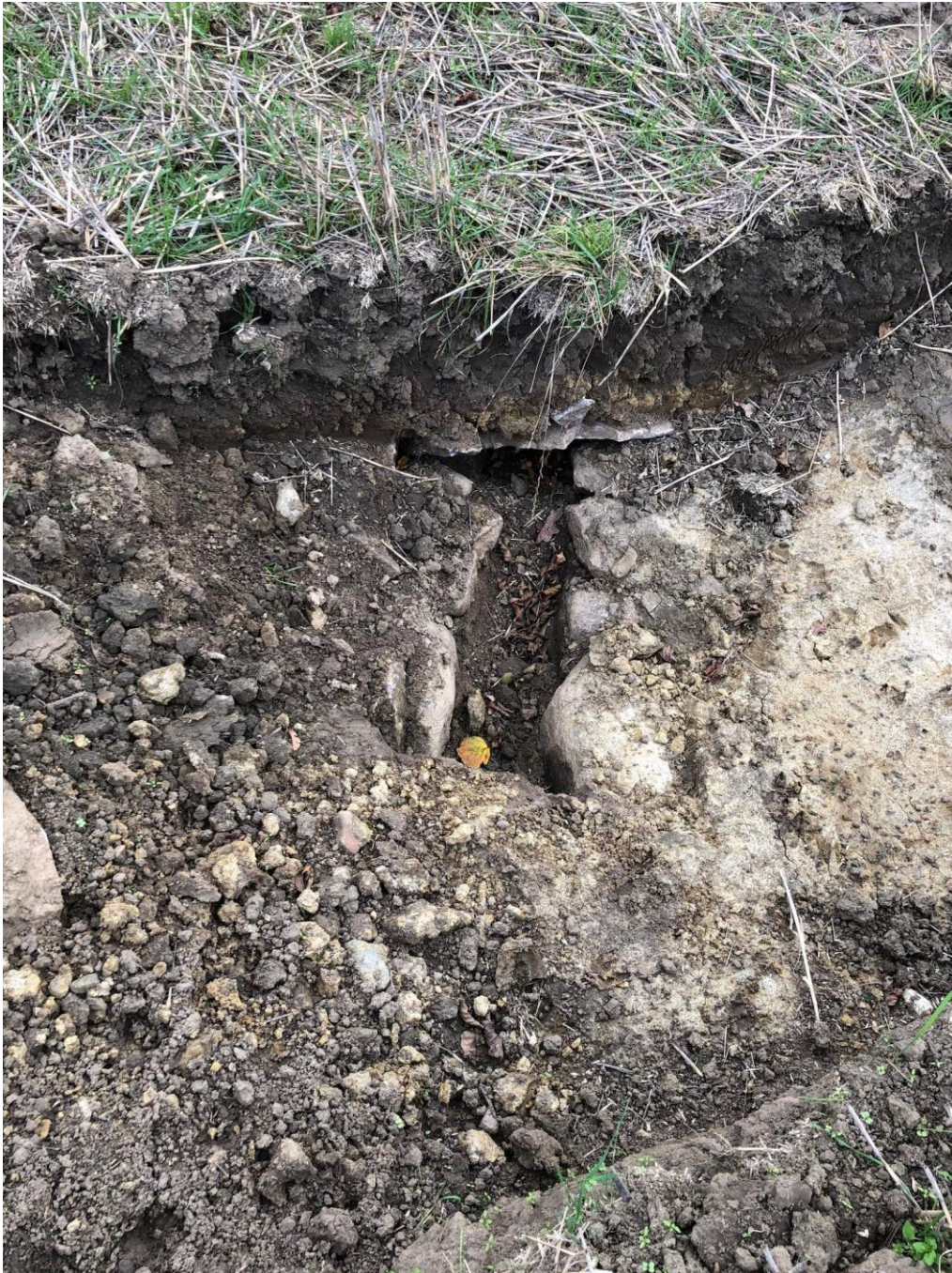
Image 5. Stone drain discovered during excavation of the North Field. The drain is still functioning.
